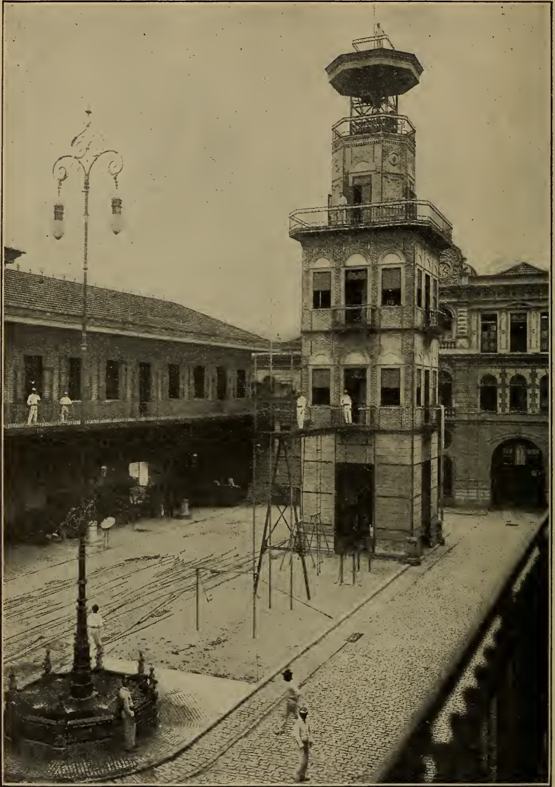
CENTRAL STATION OF THE FIRE DEPARTMENT, RIO DE JANEIRO.
